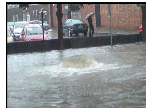
Sewer flooding Water and sewerage company
